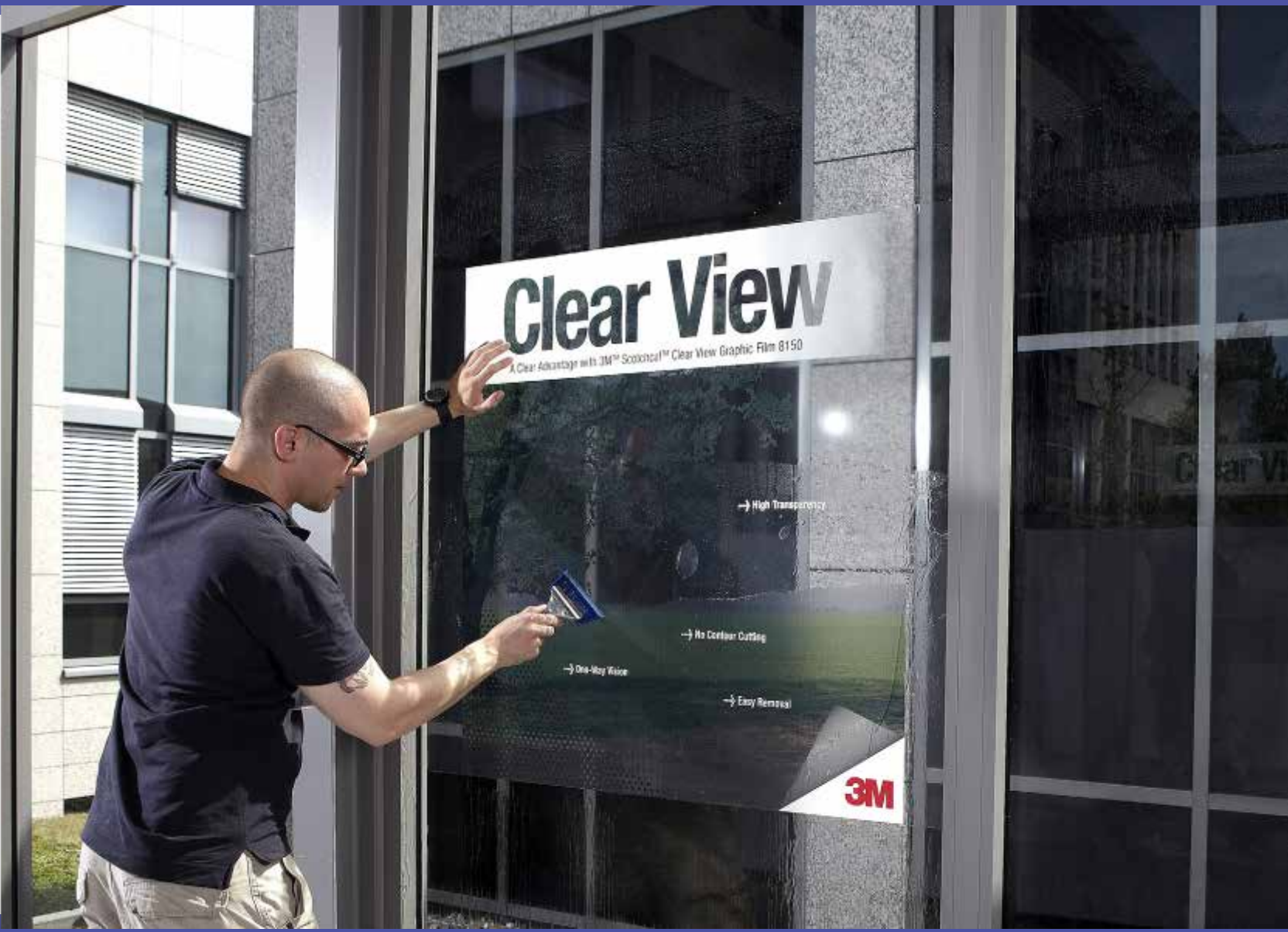
Making a perfect wet application of 3M™ Scotchcal™ Clear View Graphic Film 8150 | Step 16:
