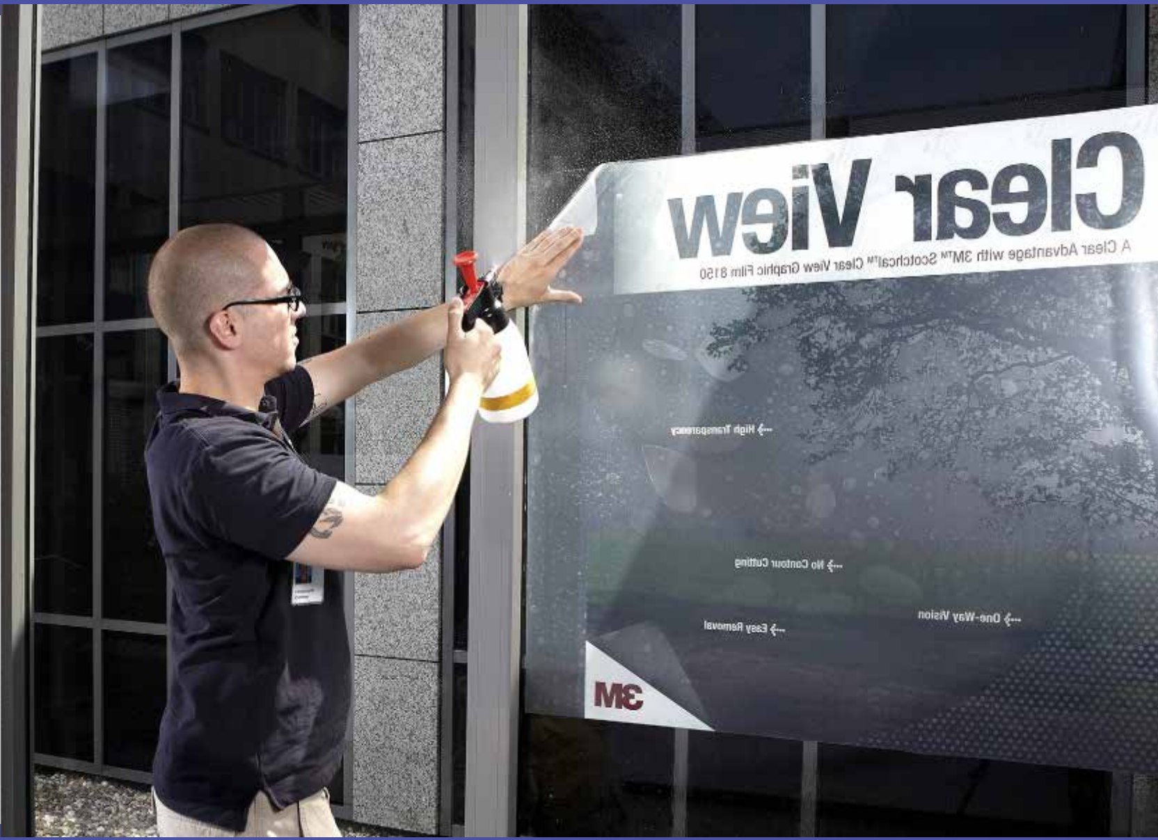
Making a perfect wet application of 3M™ Scotchcal™ Clear View Graphic Film 8150 | Step 7:
