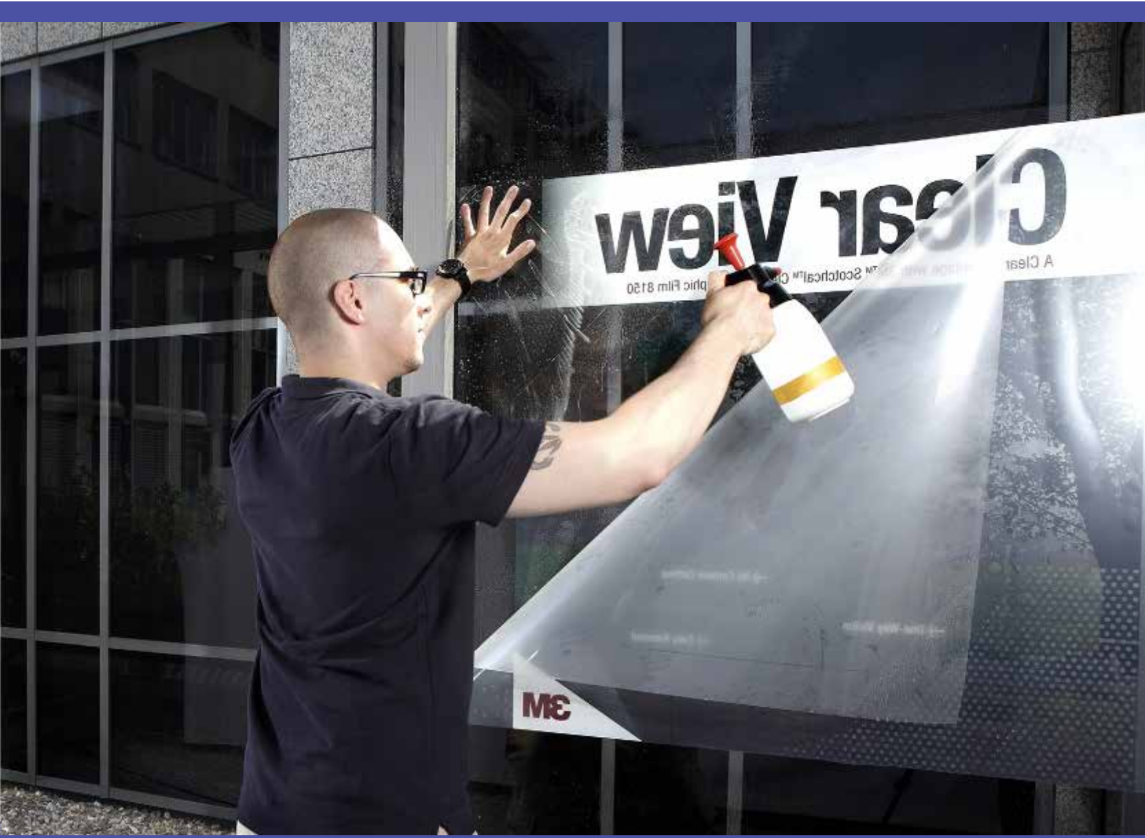
Making a perfect wet application of 3M™ Scotchcal™ Clear View Graphic Film 8150 | Step 8:
